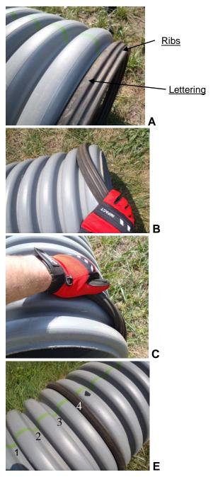
Depending on how the gasket arrives, one may need to twist the gasket so that the lettering is facing "out" and the ribs are furthest away from the pipe, figure A. Please note that this is the opposite way one would want to install the front gasket.
