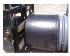
Be sure to lube both gaskets and the leading edge of the adapter. It is important not to damage the adapter during the installation. Additional end protection such as 2x4's or a wooden skid may be necessary to install the adapter. With construction equipment, push the adapter over the end of the pipe that will be installed in the MH.
