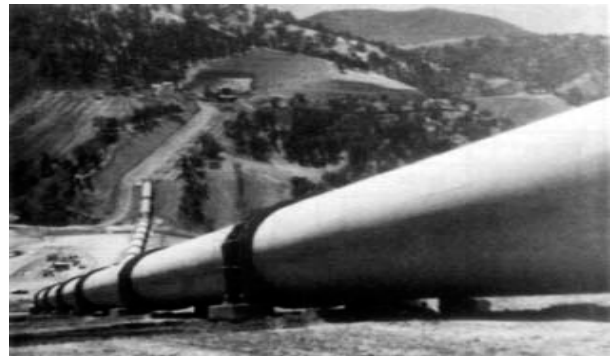
Penstock coupled with 190 inch Smith-Blair® couplings.
