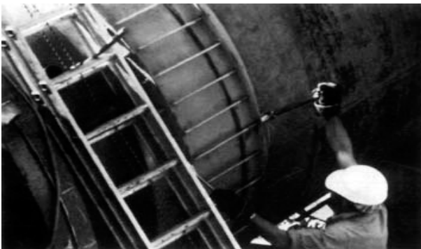
Bolting up of coupling being completed.
