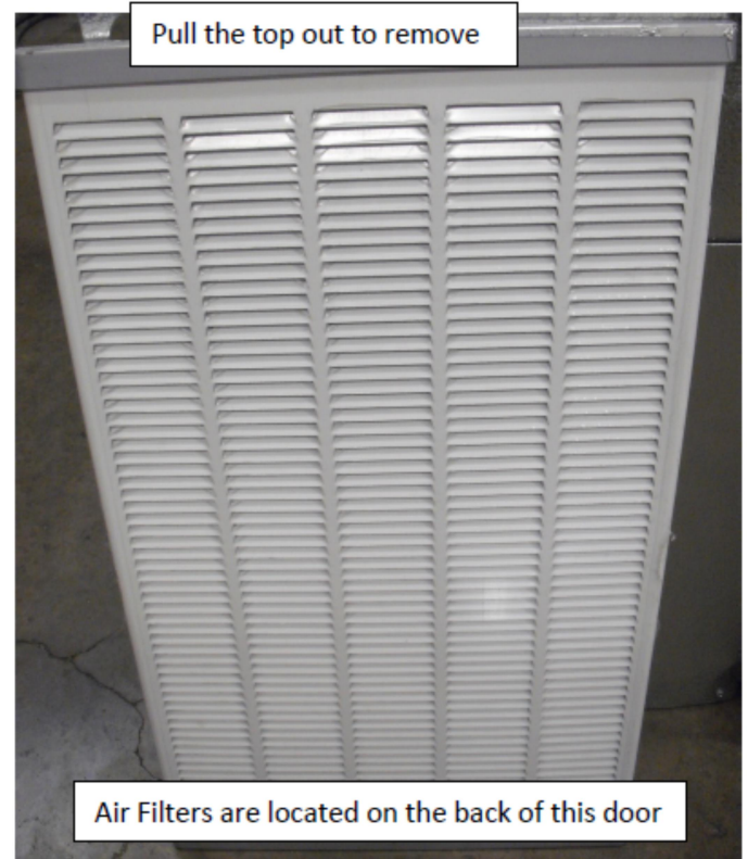
Figure 6: Return Air Louvered Door Air Filter Location
