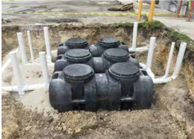
Three BIG-1150 grease interceptors installed in parallel by Bolay in Miami, Florida.
