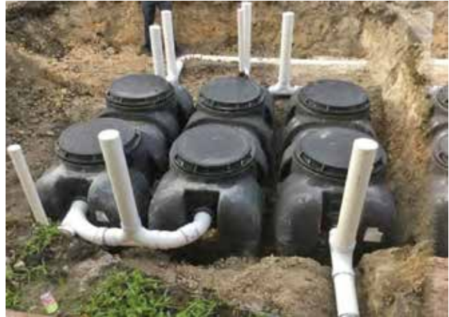
Three BIG-1150 grease interceptors installed in parallel by Bolay in Miami, Florida.
