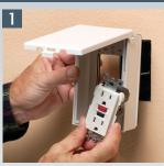
Feed device through opening (cover is removable for easier access).
