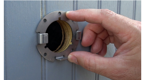
Step 4: Tab with hole positioned at 6 o'clock
