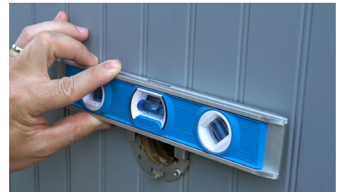
Step 4 cont'd: Ensure mounting bracket is level
