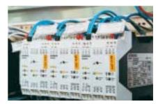
Fig. 6/3 Safe shutdown and muting using the space-saving evaluation devices with muting function
