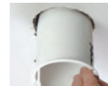
Insert housing into position and align slots in housing wall with indicator label on inside of plaster frame opening (bottom of cam lock spring blades should be positioned on flat area of the plaster frame). Then secure in position with cam locks.
