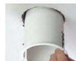
Insert housing into position and align slots in housing wall with indicator label on inside of plaster frame opening (bottom of cam lock spring blades should be positioned on flat area of the plaster frame). Then secure in position with cam locks.
