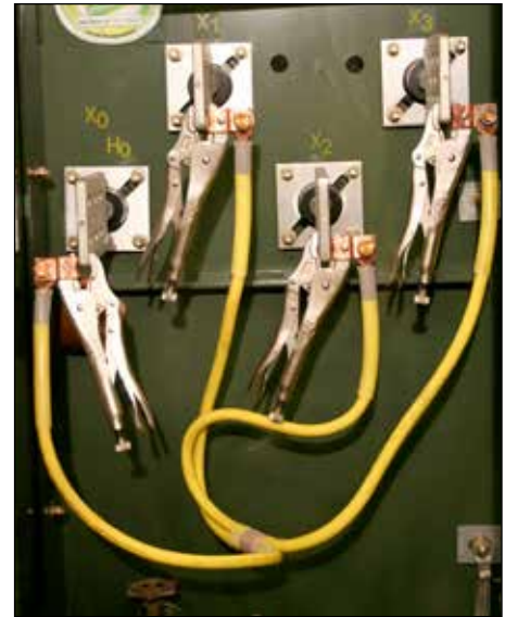
Figure 23. Applied to transformer secondary.
