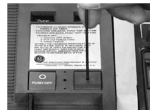
Activating the breaker closing mechanism through the hole in the Hidden "ON" Button
