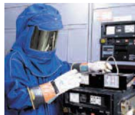
NEC Handbook Exhibit 110.7 Electrical worker clothed in personal protective equipment (PPE) appropriate for the hazard involved 1 .
