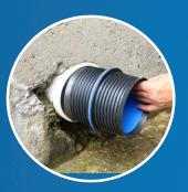
**Step 2**Lubricate gasket O.D. with soap & water solution
