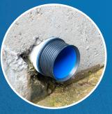
**Step 3**Push in place up to the pipe stop
