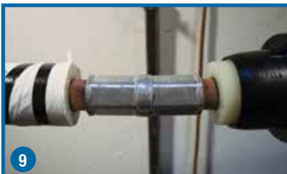
9 Conductors shown joined using a compression connector.
