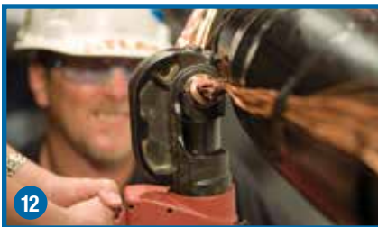
12 Connect neutral wires as required.
