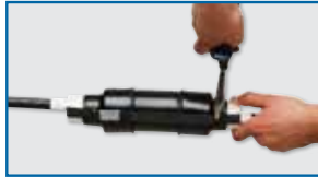
Cut fastening straps.
