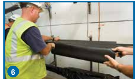
6 Store the cover-up sleeve on each cable.
