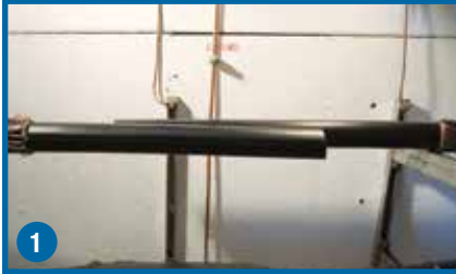
1 Overlap cables, straighten and strip back jacket.
