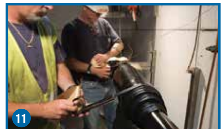
11 Seal joint ends with mastic wrap.
