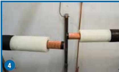
4 ...and bare the conductor.
