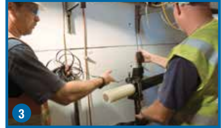
3 Remove the semi-conductive shield...
