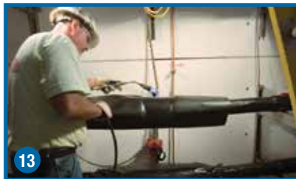
13 Position and shrink cover-ups.
