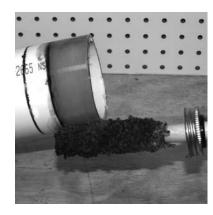
without re-dipping the applicator in the cement, apply a medium layer of cement to the fitting socket aggressively working it into the surface. On bell end pipe do not coat beyond the socket depth.
