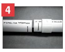
coupling has raised quarter mark lines on the outside diameter of the coupling.)
