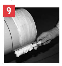
Apply a medium layer of cement to the fitting socket aggressively working it into the surface. On bell end pipe do not coat beyond the socket depth.
