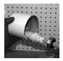
Apply a second coat of primer to the fitting socket aggressively working it into the surface.
