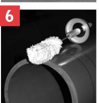
Too small an applicator will not apply sufficient cement.
