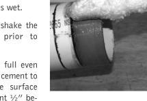
yond the hub depth. Aggressively work the cement into the surface.
