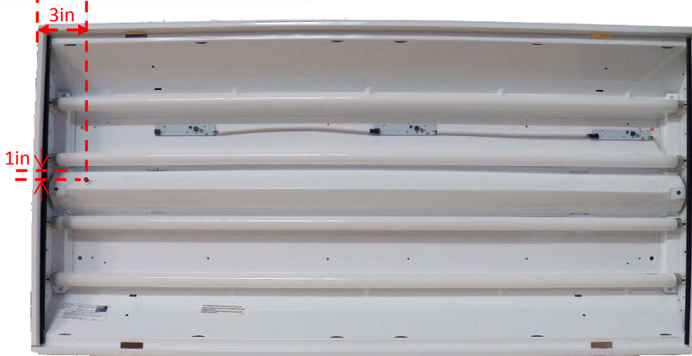
Example of 2X4 Troffer with completed installation and wire way reattached
