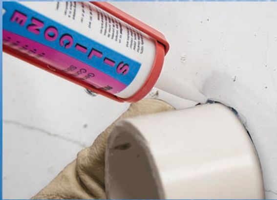
Seal wall opening with 100% silicone caulk.
