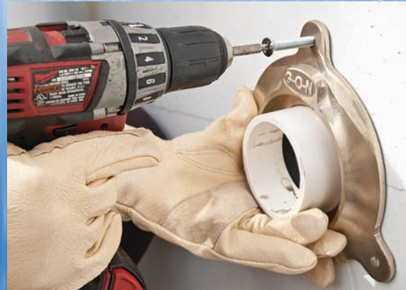
Install anti-theft escutcheon & secure with appropriate anchor.
