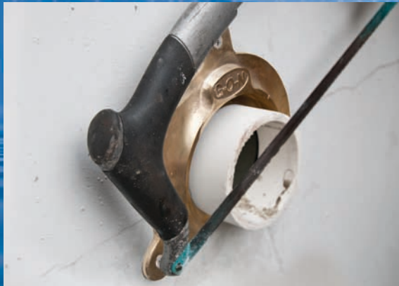
Measure hub depth of G-O-N & cut stub-out to proper length.
