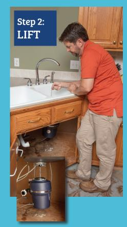
Raise the disposal up through the drain opening until it engages the sink flange. Then apply tension to the spring.
