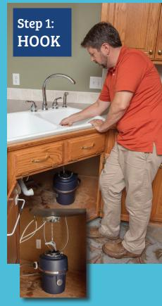
Drop the hook down through the drain opening into the disposal, then pull up to center it inside the grinding chamber.
