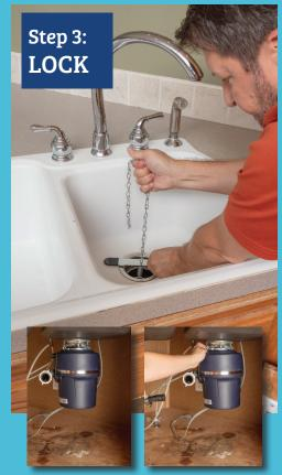
Slide the chain into the locking bar, maintaining the tension on the spring, then let go. The disposal is now secure for you to reach under the sink and engage the locking collar with EASE!
