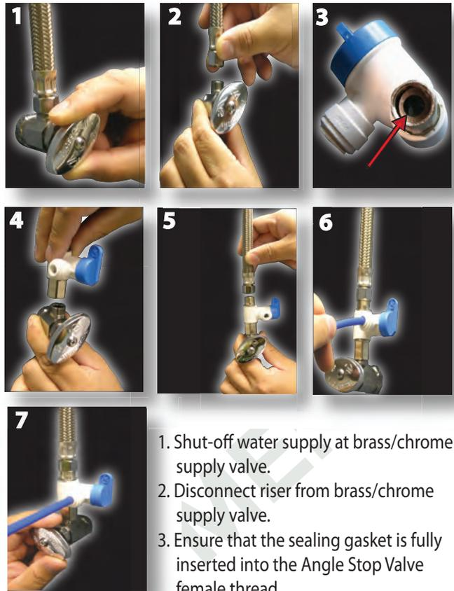
1. Shut-off water supply at brass/chrome supply valve.
