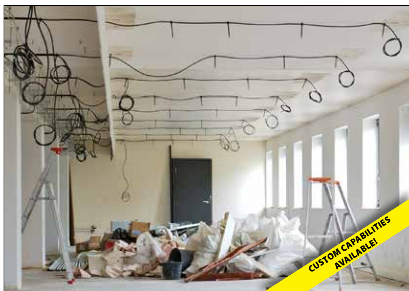
Custom made “powered” Drop Cords for a newly renovated commercial office building.
