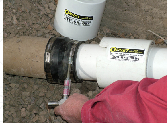
Step 2 Attach flexible coupling to pipes making sure clamp screws are aligned before tightening both bands.
