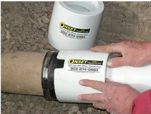
Step 3 Slide Shear Guard™ into place over flexible coupling aligning clamp screw into key hole.
