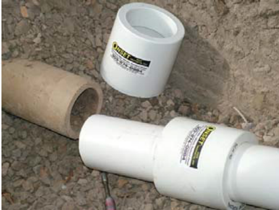
Step 1 Slide the Shear Guard™ support onto exposed pipe that is to be joined to existing pipe.
