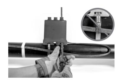
**5.** Ensure min. 9" (229 mm) remains for cable termination and tape service loop.
