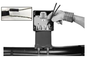
14. Feed field wiring power and ground conductors into the cutout in junction box using suitable wiring method. For hazardous location installations the wiring method shall comply with one of the wiring methods permitteed in the NEC or CEC (as applicable) for hazardous location classification of the installation. Ensure the grounding conductor and raceway used for field wiring are grounded on the grounding plate inside the junction box
