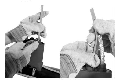
**8.** Wrap tape around the braid 1" (25 mm) from end of the outer jacket cut back.
