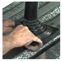
WRAP... Wrap Retro-Fit around pipe and install all snap rivets to seal flange.
