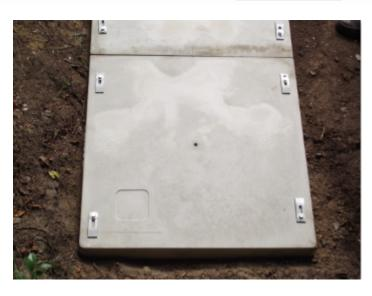
Set the pad halves on flat, packed ground or with a bed of sand below it.
