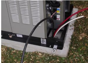
Guide lines in the GenPad LC ensure that the generator will be positioned perfectly the first time
