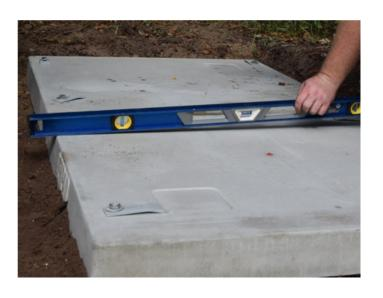
Ensure that both pad halves are level.
