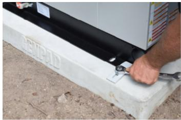
Secure the frame of the generator into the inserts within the GenPad LC
