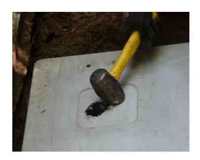
Use the knockout which matches the location where cabling runs into the generator
