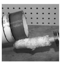
• Remove excess cement from the exterior. A properly made joint will show a continuous bead of cement around the perimeter. If voids appear sufficient cement may not have been applied and joint failure may rocult.
