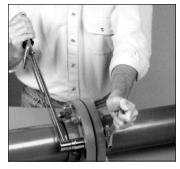
8. When installing flanges in a buried application where settling could occur, the flange must be supported to maintain proper alignment in service.
