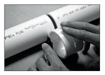
4. Place the repair coupling on the pipe with the larger pipe ID (inside diameter) end facing the gap between the pipe ends. (The larger pipe ID of the
