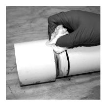
Align all piping system components properly without strain. Do not bend or pull pipe into position after being solvent welded.
