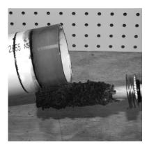
Without re-dipping the applicator in the cement, apply a medium layer of cement to the fitting sockaggressively working it into the surface. On bell end pipe do not coat beyond the socket depth.
