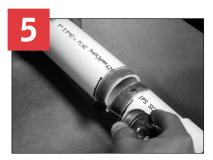
Apply heavy body cement between the mark and pipe end on both pipe ends.
