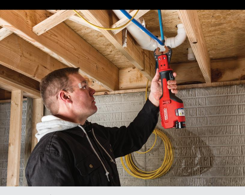
The RIDGID® PEX-One™ 12V Battery PEX Tool is designed for contractors who repair or install PEX plumbing systems. The lightweight, low-profile PEX-One presses multiple-size connections, up to one inch, with a single tool. The RIDGID PEX-One gives you the one-handed functionality you need for easy and accurate press connections in tight or hard-to-reach spaces.
