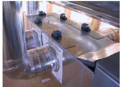
Customize plenum opening to transition to coil or air handler. Seal and insulate per local code requirements.
