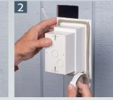
Apply the supplied caulk around back edges of flange. Install NM cable connector and wire, then press onto surface.
