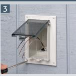
Attach IN BOX with stainless steel screws (provided).
