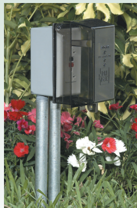
Why install boxes this way...
