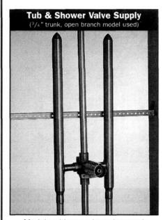
Models with open branches work great for tub valve connections.
