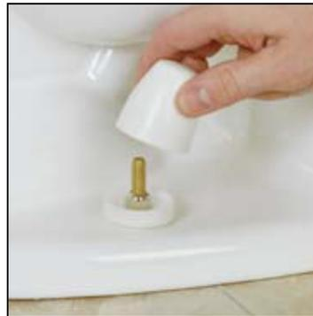
Base is installed between the bowl and nut.
