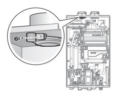
5. Pull the filter out of the water heater.
