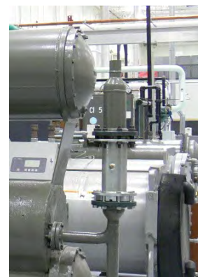
Figure 18. Rupture Disc.
