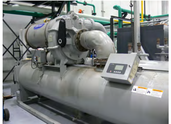
Figure 17. Low-Pressure Chiller.
